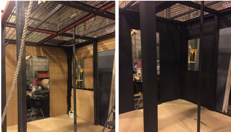
Subway car before (L), primed in Rosco Tough Prime Black (R) notice how consistent the finish is despite three different substrates
